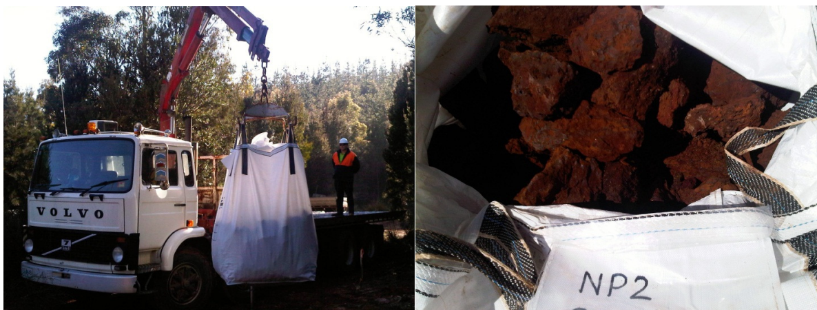
Figure 1 – Barnes Hill ironstone material being shipped for beneficiation
